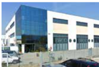
Engineering & Training Center
