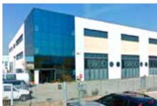
Engineering & Training Center
